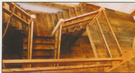
Stairs are made of 2-inch oak planks.
