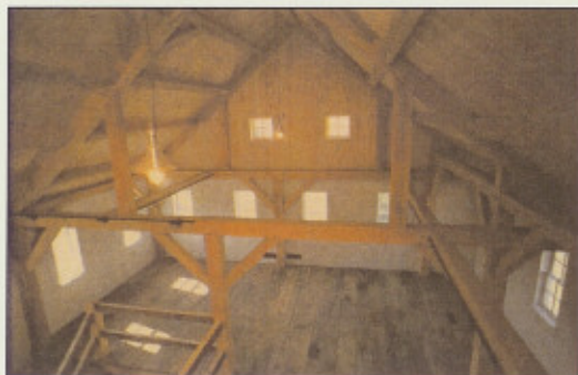
A view of the loft reveals the barn's simple structure.
